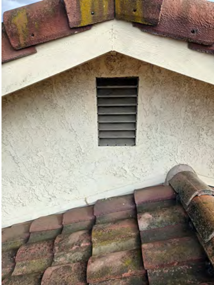
Attic and garage vents with 1/16" screens installed by Blaze Blockers.
